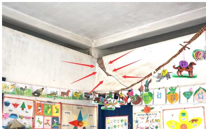
Figure 2: The wall crack in Mitaapheap SPS
