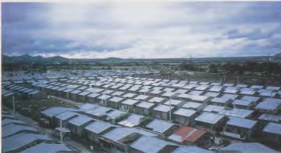
Photo1 Low-Cost Housing/ Calamba
