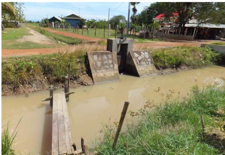
Photo 1 Water gate along the main canal in Bos Ta Ney Village
