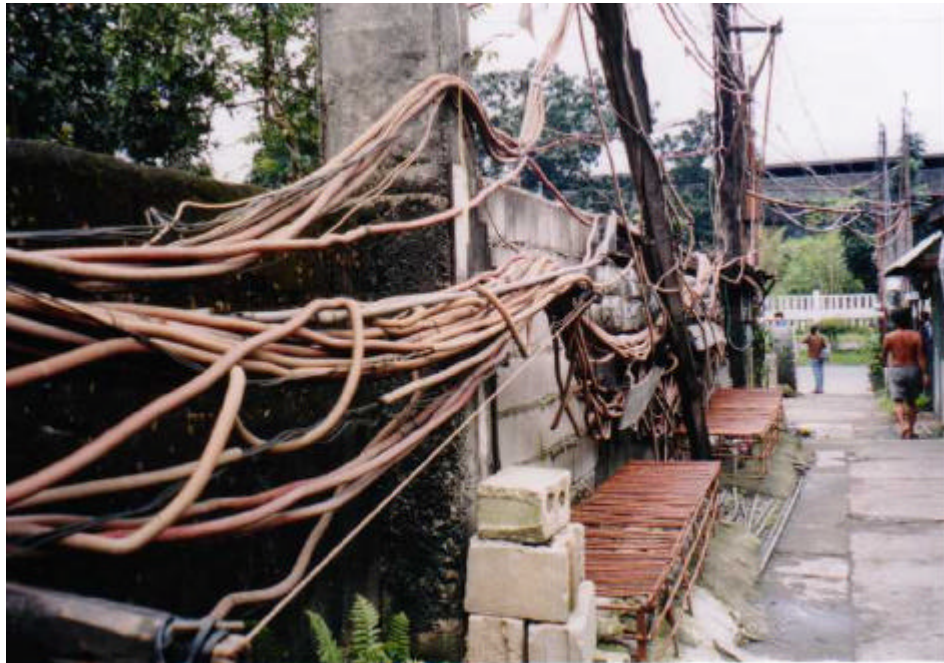
Picture 2: Spaghetti connections of electricity (upon the wall) and water (on the ground) in Manila
